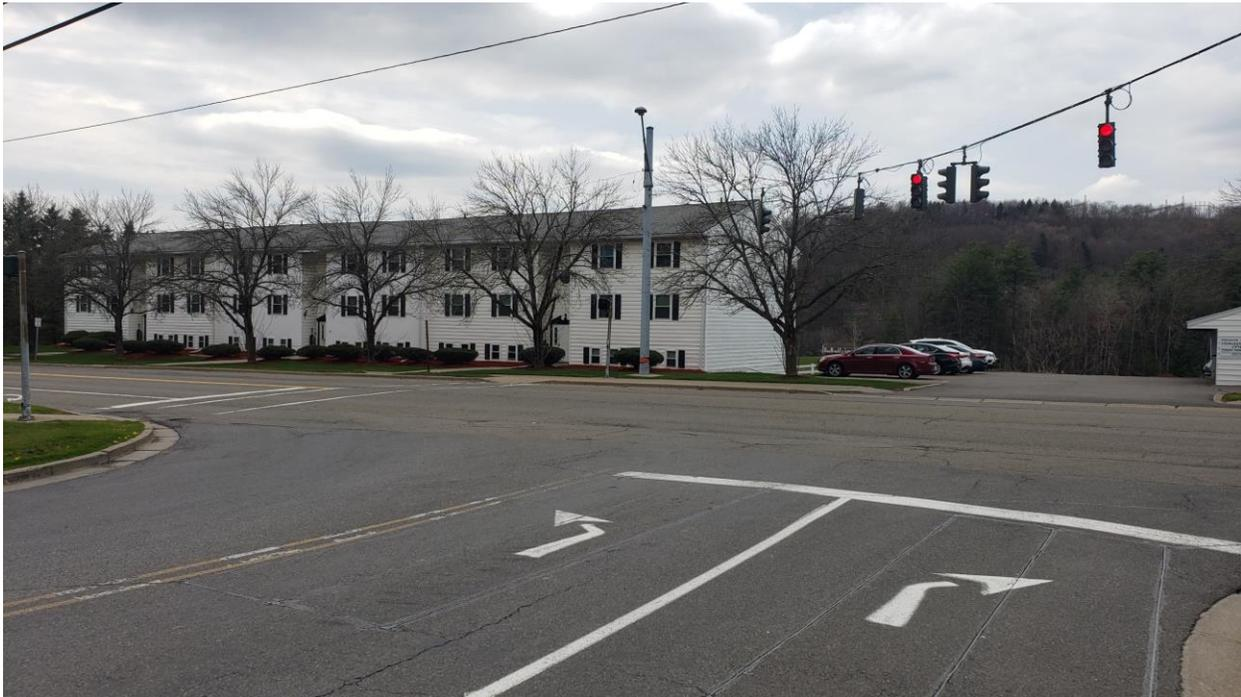
This signal was installed because it is at the entrance to the Johnson City School Complex that includes it's elementary, middle and high school. The signal is actuated with pedestrian signals. The pedestrian signals are old, and the walk symbol illumination is not very bright. These should be replaced with count down pedestrian signals with upgraded ADA curb ramps and high visibility crosswalks.
