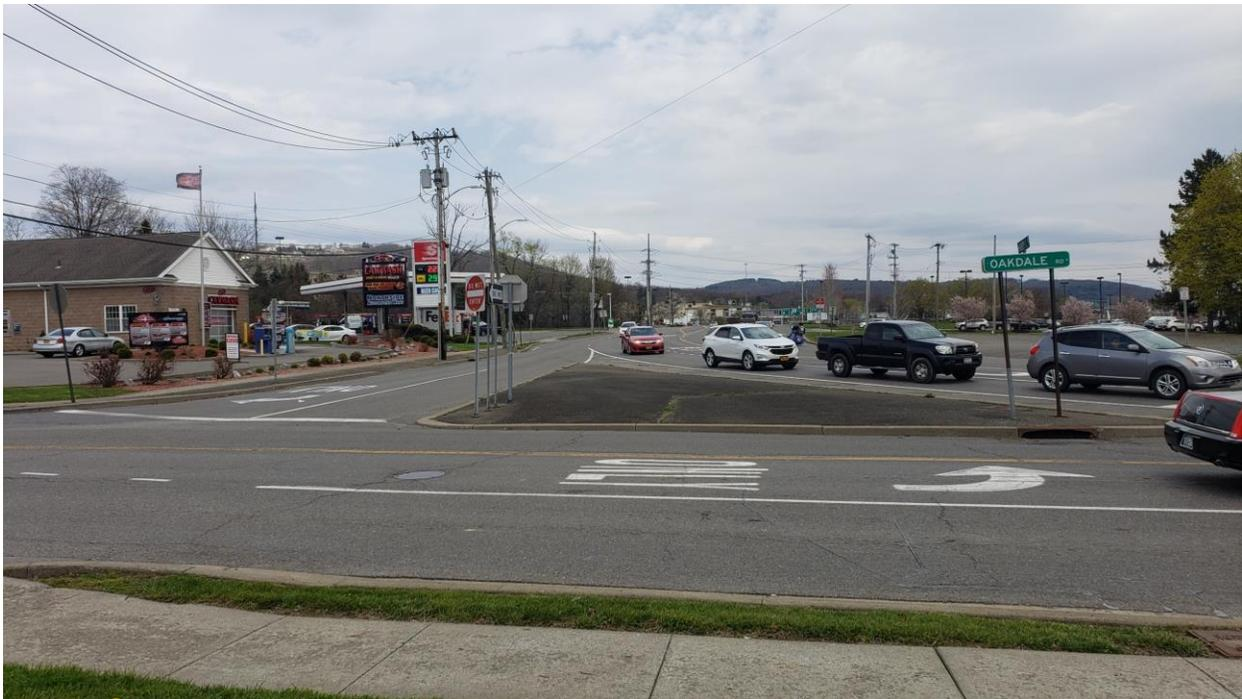
Harry L. Drive and Oakdale Road is a four-legged intersection but does not have the typical configuration. The westbound right turn is stop sign controlled and separated by an island from the signalized portion of the intersection. This intersection, while not totally meeting the signal warrants, does come close to the volume warrants, and while not meeting the accident warrant
