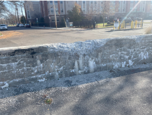
Photo 1: Binghamton- Floodwall deteriorating at Water and Susquehanna Street
