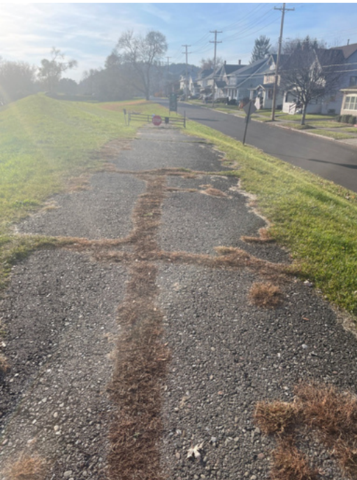
Photo 12: Endicott Chugnut- Cracking and overgrowth near River Terrace
