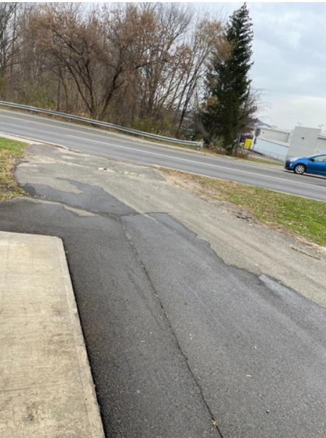
Photo 10: Vestal Rail Trail- Cracking and depressions at east entrance by African road
