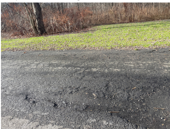
Photo 6-8: Otsiningo- Cracking and Puddling on north end of trail
