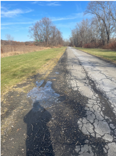
Photo 6-8: Otsiningo- Cracking and Puddling on north end of trail
