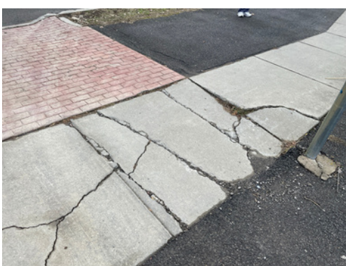
Photo 3: Binghamton- Cracking and pavement changes above East Clinton
