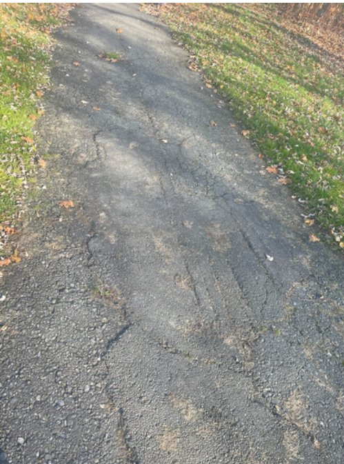
Photo 14: Endicott Chugnut- Severe Cracking behind school
