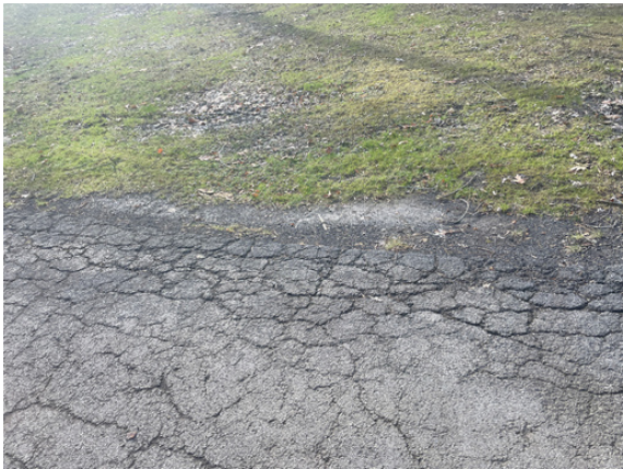
Photo 9: Port Dickinson- Severe Cracking at northmost end of the loop
