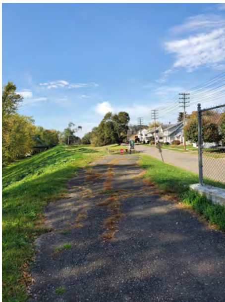
Photo 16. Endicott I Vegetation encroachment onto the trail and pavement
