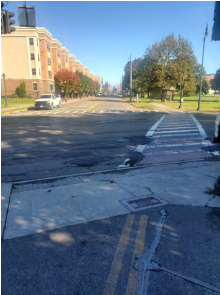
Photo 1. Binghamton | Curb ramp at the Intersection of the S. Washington Bridge Entrance and Route 363 in poor condition
