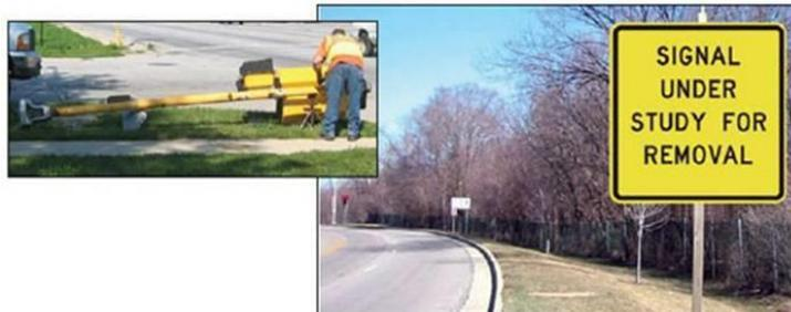
3. Covered Signal Evaluation - Following the installation of required traffic control signs and road markings, an evaluation period of 90 days or longer will be utilized to assess impact on traffic flow. An alternative procedure for the 90 day period may include a flashing period for part or all of the 90 day evaluation. The flashing configuration will reflect either a four way or two way stop.
