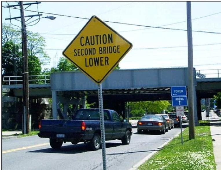
Figure 4.5 12'-1" Clearance Sign on Railroad Overpass over Front Street
