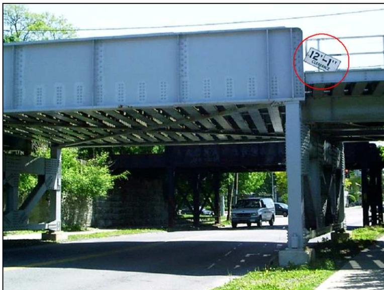
**Figure 4.6 12'-1" Clearance Posted on Opposite Approach to Front Street Railroad Overpasses**
