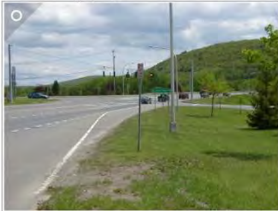
Rural signalized intersection, with shoulders for vehicular turns.
