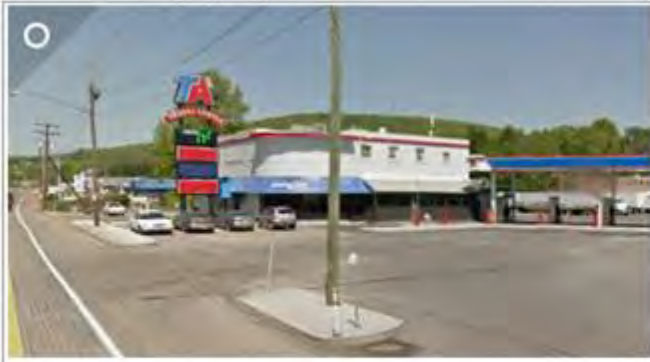
Gas station with multiple wide curb cuts, easy access for vehicles, no landscaping or areas for drainage.
