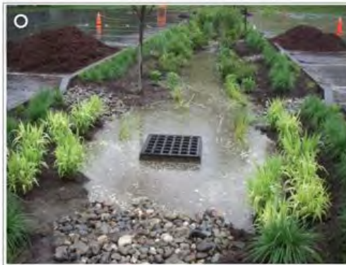
Defined curbs that allow stormwater to flow and filter into a natural drainage area and away from the street and parking lot. Some maintenance required but localized flooding reduced.
