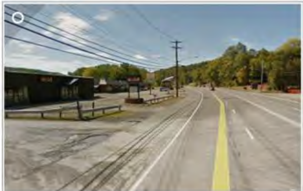
Four vehicle travel lanes and wide shoulders (faster traffic speeds), no landscaping, little maintenance required.
