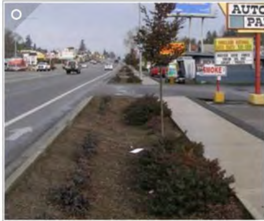
Same street, with defined driveways that restrict street access but reduce conflict points between vehicles and pedestrians, sidewalks and landscaping.
