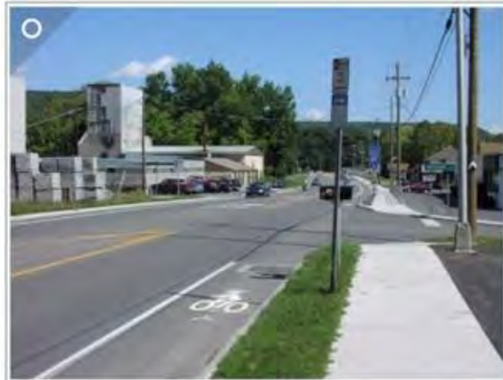
Same street with narrower vehicle lanes (slower traffic speeds), center turn lane, bike lanes and sidewalks
