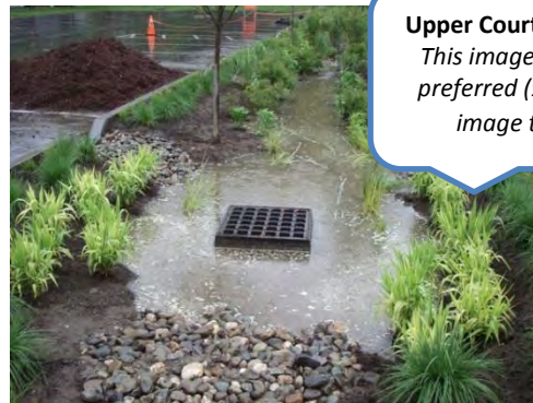
Image 3.4: Bioswale collecting water from a parking lot.
