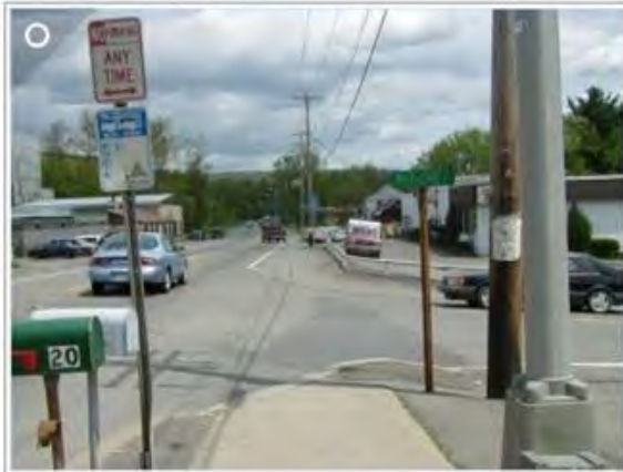
Street with wider vehicle travel lanes (faster traffic speeds), limited or no areas for pedestrians and bikes
