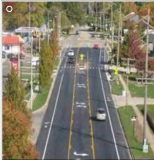
Two vehicle travel lanes (may slow traffic), center turn lane (reduces turning conflicts), bike lanes, mid block pedestrian crossing.
