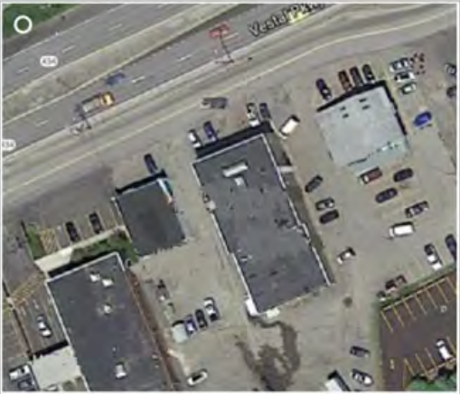
Cars may access business from anywhere along street, no landscaping, safety impacts from cars backing into street.
