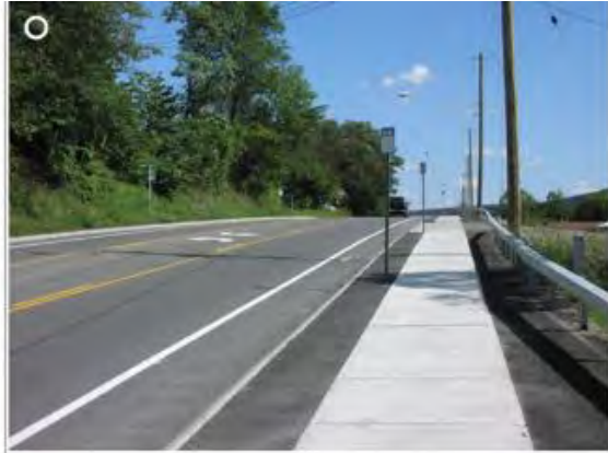
Same roadway with center turn lane, bike lane and sidewalks.
