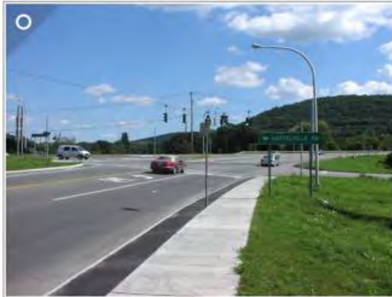
Same signalized intersection with sidewalks and more restrictive areas for vehicle turns.
