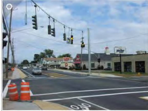
Same street with defined curbs, sidewalks and bike lines, more restrictive vehicular access and narrower travel lanes.
