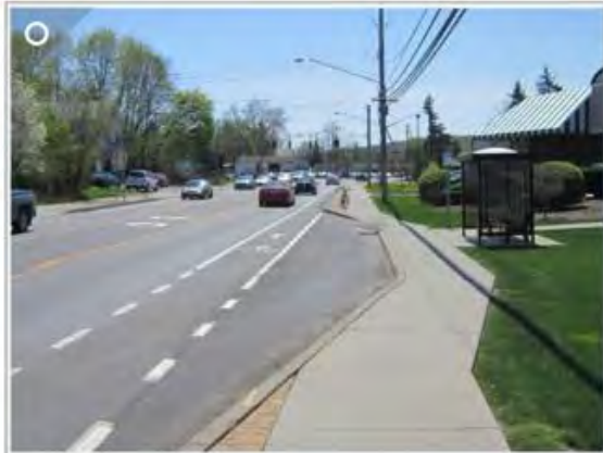
Defined bus pull out and sheltered bus stop, sidewalks and bike lanes.
