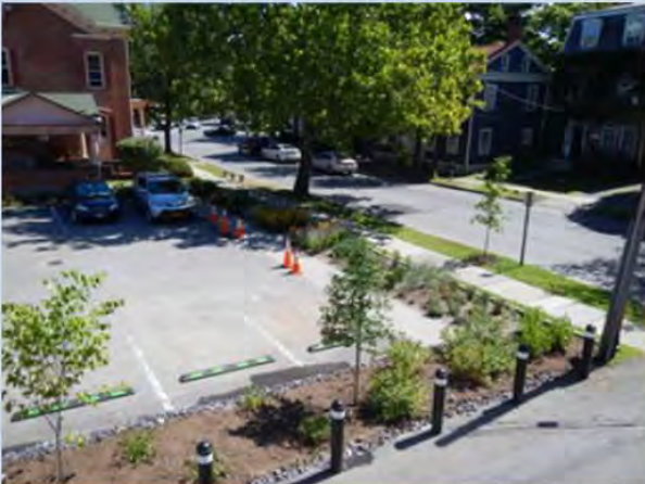
Parking lot after installation of green infrastructure
