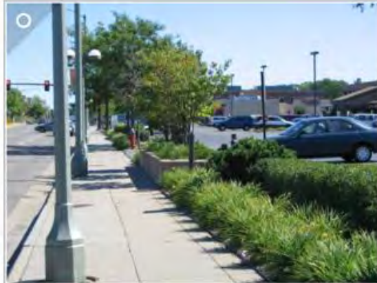
Street Facing parking lot, landscaping requiring maintenance, sidewalks and decorative lighting.
