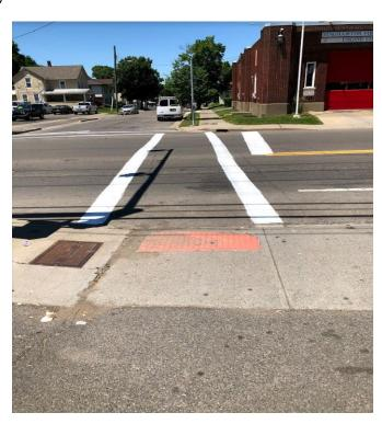
the westside of Broome Street. This will provide a safer crosswalk location and move it out of the driveway on the southside of Conklin Avenue. Bike lanes need to be repainted with the bicycle symbol placed within the bike lanes from Broome Street to Baldwin Street. The school speed zone sign should have a yellow S<sub>4</sub>-3 school sign.
