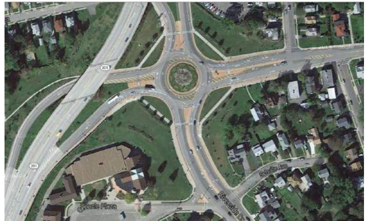
Two lane roundabout with surrounding shared-use path in Johnson City, NY
