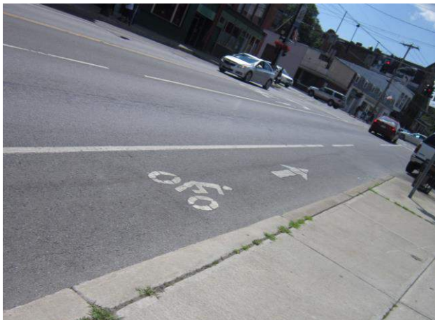
Bicycle lane on Court Street Bridge, Binghamton, NY
