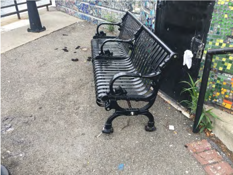
Figure 35 Bench Bent Out of Place
