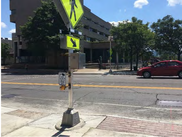
Figure 36 New Court Street Crossing
