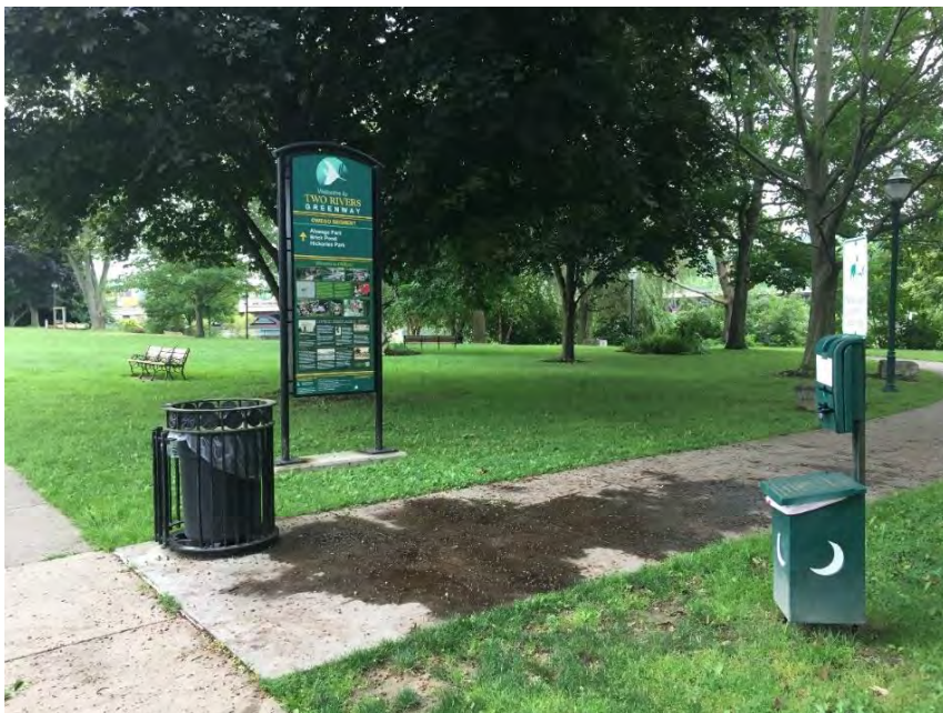
Figure 68 Puddling from Overhanging Trees
