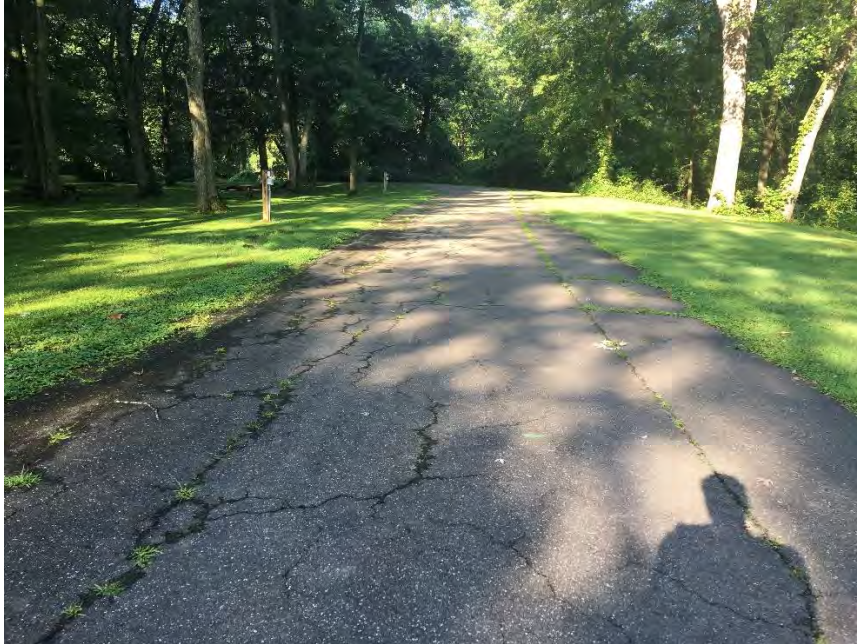
Figure 73 Cracked Pavement
