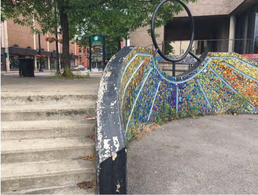
Figure 32 Worn Paint and Weeds Along the Edges
